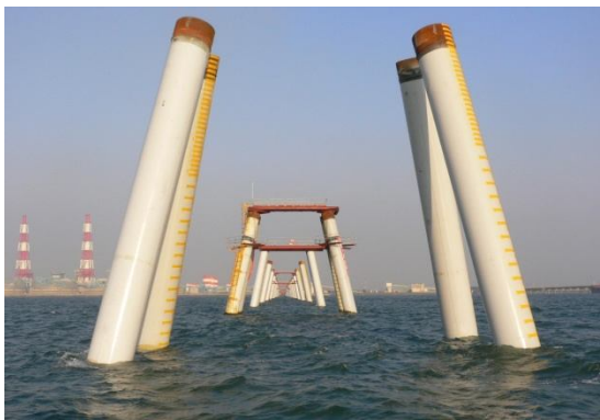
Hangzhou Bay Bridge, Hangzhou, China Length 89m diameter 1600mm Thickness 15-18mm
