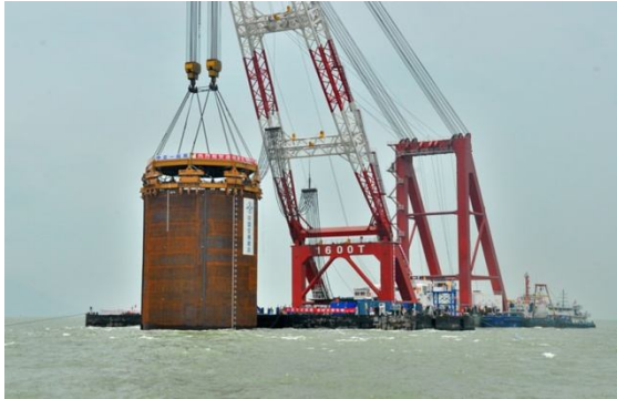
China South Sea Project Diameter:21m Length:85m Weight:705tons/pipe
