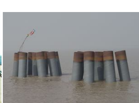
NIMR-G Development West Water Flood Project, Oman 42"x11.13mm 45m
