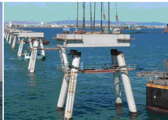
Hangzhou Bay Bridge, Hangzhou, China Length 89m diameter 1600mm Thickness 15-18mm
