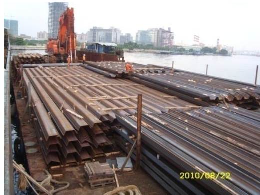
Sheet Pile Shipment
